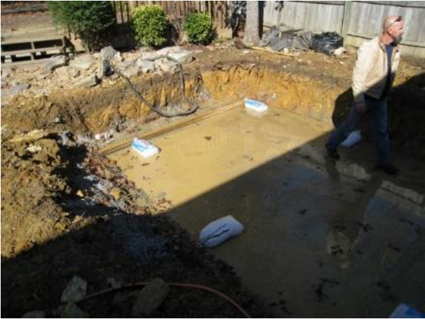
Figure 7. Ice Bag Positioning in Excavation
