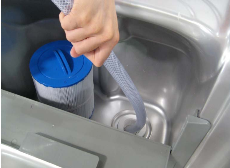
Figure 8. Filling Location in Filter Housing
